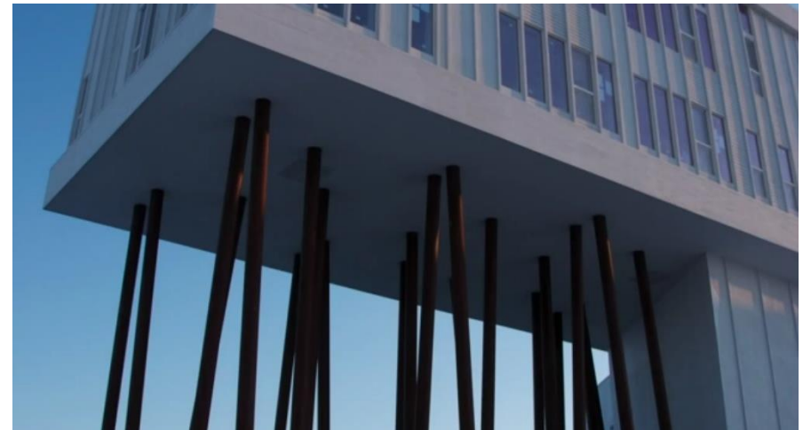
Figure 6 - Another view of the stilts and overhang
