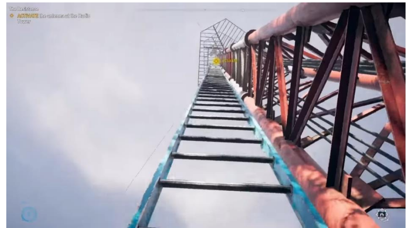
Figure 11 - appearance of tower from base
