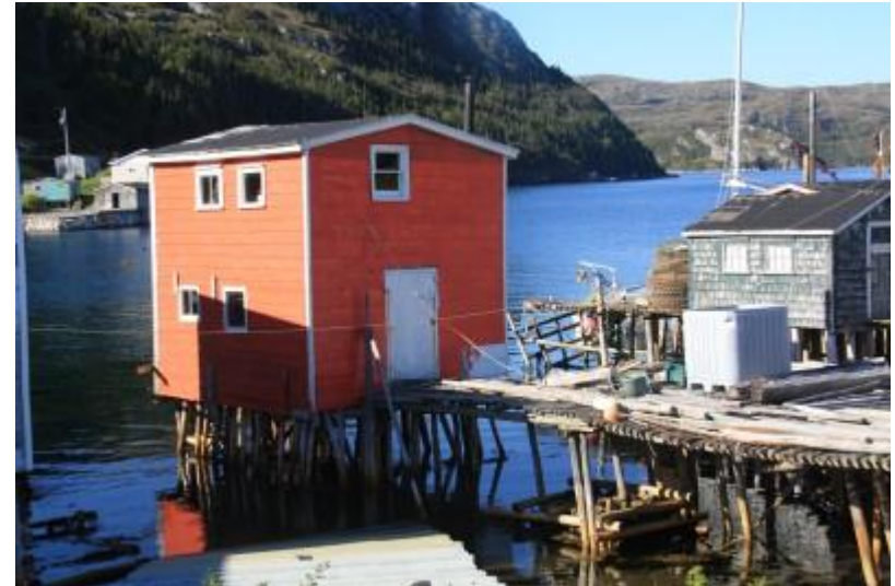
Figure 7 - a mundane building on stilts, which the inn can follow after
